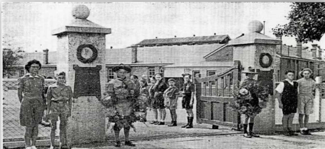
THOMAS STREET STATE SCHOOL MEMORIAL GATES Laying of Wreaths on Anzac Commemoration
